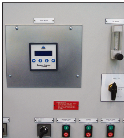
Installation of the AAL7000
